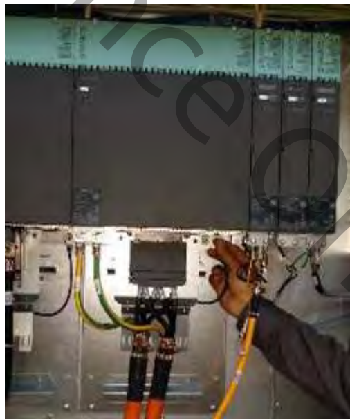
Figure 5-154: Connector Disconnect from Latch
